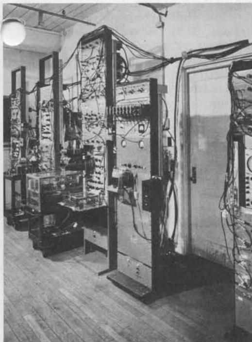
**Pulse Testing.** A sample of 50 cores from each lot was used for hysteresis-loop measurements. The test equipment for pulse testing and semiautomatic selection testing consisted of an electronic core counter, an evaluation pulse tester, fully automatic and semiautomatic core testers, and a plane tester.
