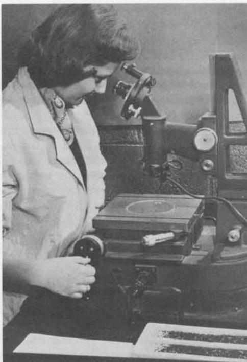
**Dimensional Check.** The machine die and the weight of the pressed cores had to be continually monitored to insure maximum uniformity of core size. Before each press run a dimension check was made with a toolmaker's microscope in order to assure quality control.
