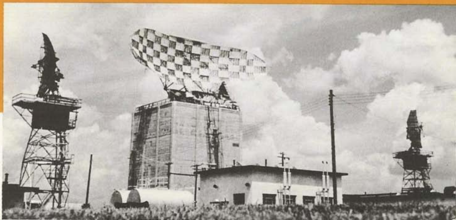
TWO HEIGHT FINDER RADARS flank a search radar at a long range radar site.
