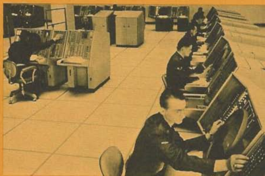
WEAPONS DIRECTION ROOM —When the air situation requires employment of air defense weapons the weapons director will select the base and type or number of weapons to be used against the hostiles or unknown. In this view, on the left is the Weapons Director and to the right are the Intercept Directors and Technicians.
