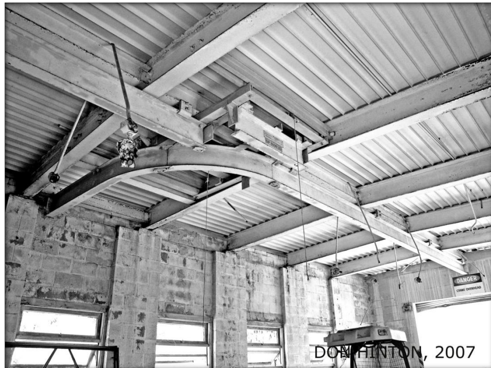
Interior of the Warhead Assembly Building at OA-63L showing overhead trolley to lift warheads. Don Hinton
